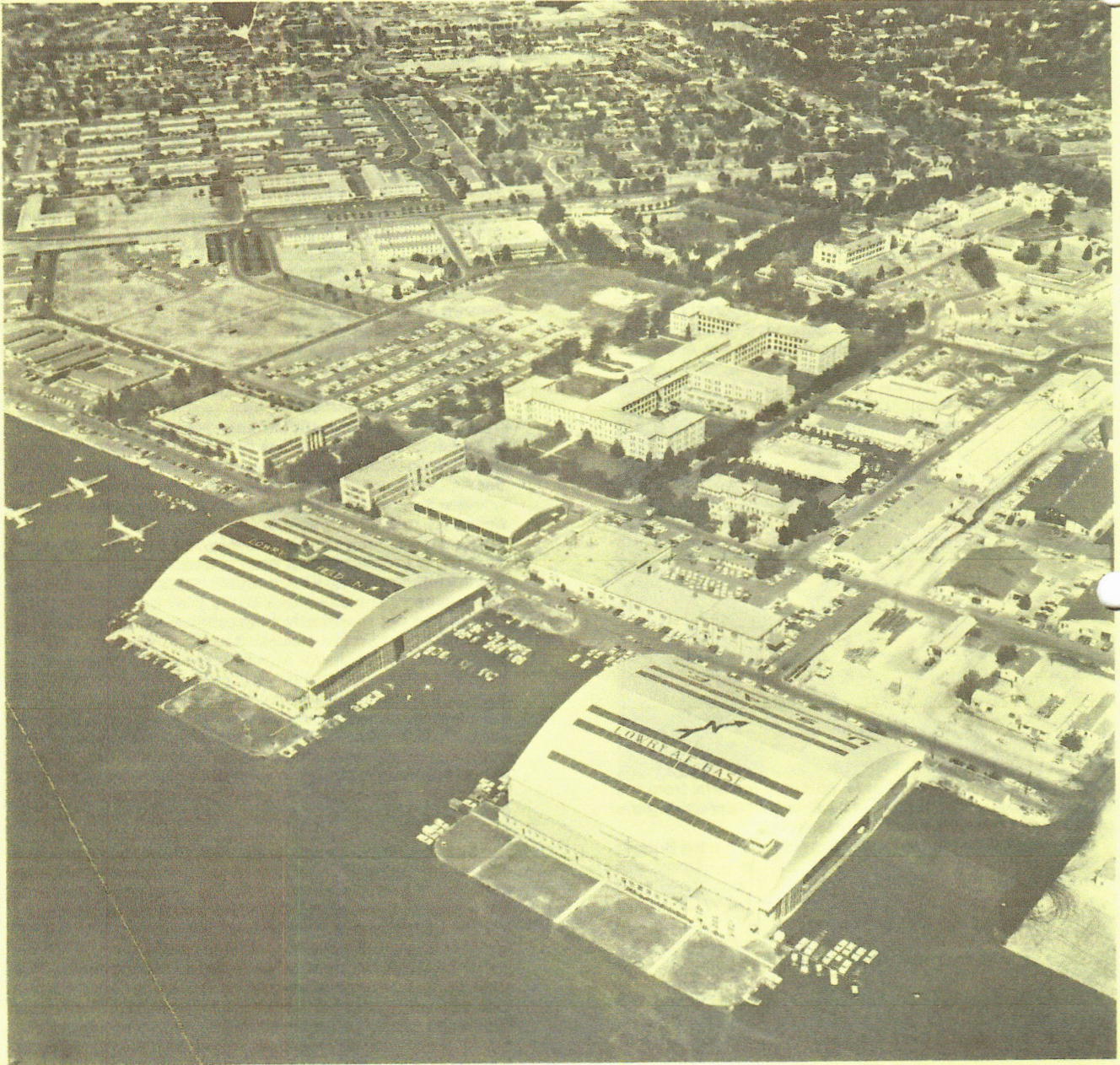
Lowry Air Force Base, 1960. Left side of picture is south; right side, north; top, west; and bottom, east.
